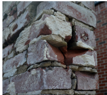
Mortar is incompatible with historic masonry when it is too hard and causes brick spalling and breakage.
