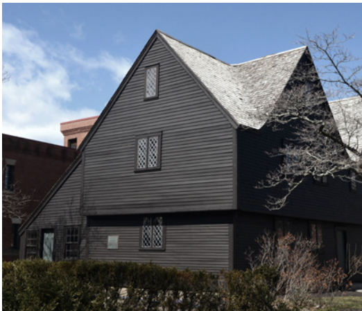
Wood shingle roofs are found on Salem's early buildings, like the John Ward House representative of the First Period style.
