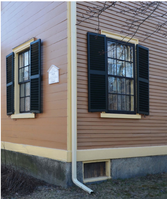
Different types of wood siding at a primary facade and secondary facades is common, like this house with flush boards (left) and clapboards (right).
