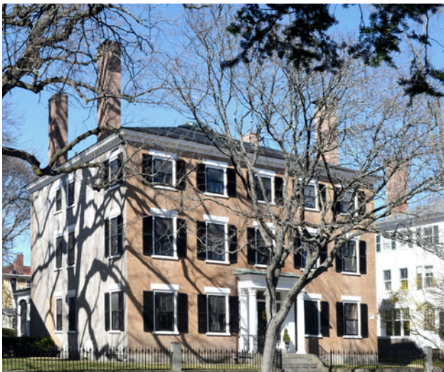
High-style Federal buildings feature symmetrical interior chimneys, creating distinctive rooflines and streetscapes in a district.
