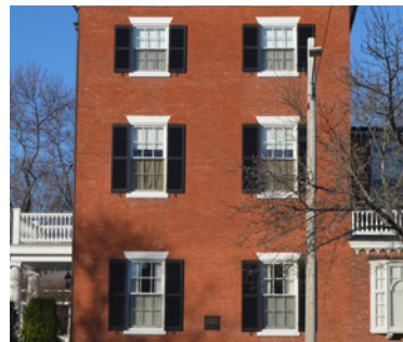
Example of 6/6 double-hung windows, a common type throughout Salem.
