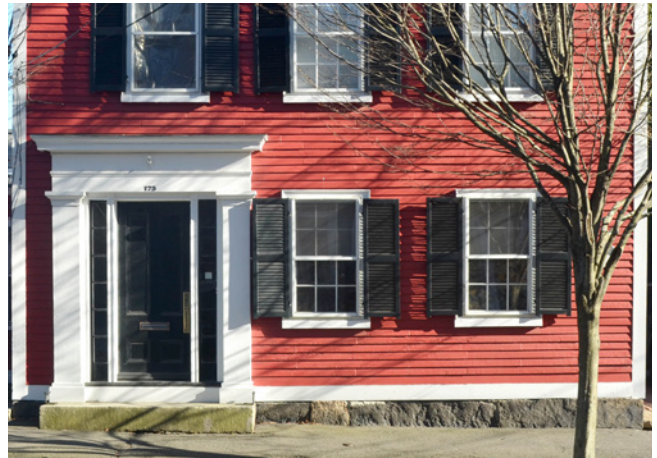
Greek Revival door with wide flat entablature and pilasters, rectilinear sidelights, and off-center/side-hall facade composition.
