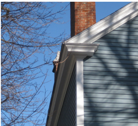
Eave moldings are essential features to consider when replacing or installing a gutter or downspout. Existing trim should be retained and the profile of the gable return should remain intact.
