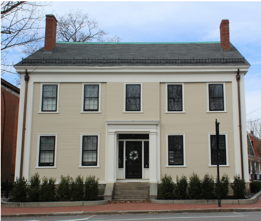
A recently restored residence in the Washington Square Historic District.
