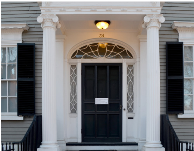
Federal door with elliptical fanlight and sidelights with tracery and columned portico.
