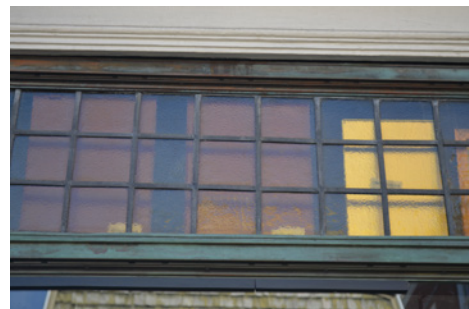
Historic transom glazing and storefront framing should be retained and restored.
