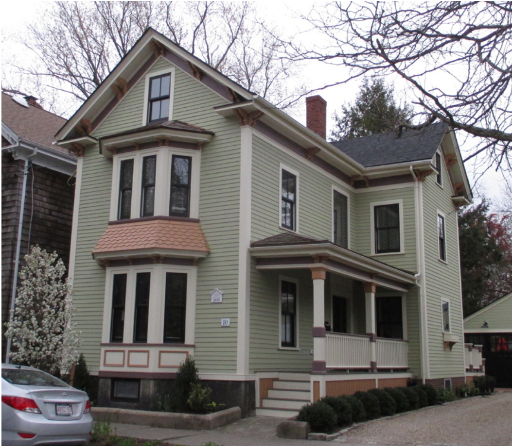
A recently restored house in the McIntire Historic District that showcases historic wood, including Italianate double brackets and Queen Anne-influenced bay window.
