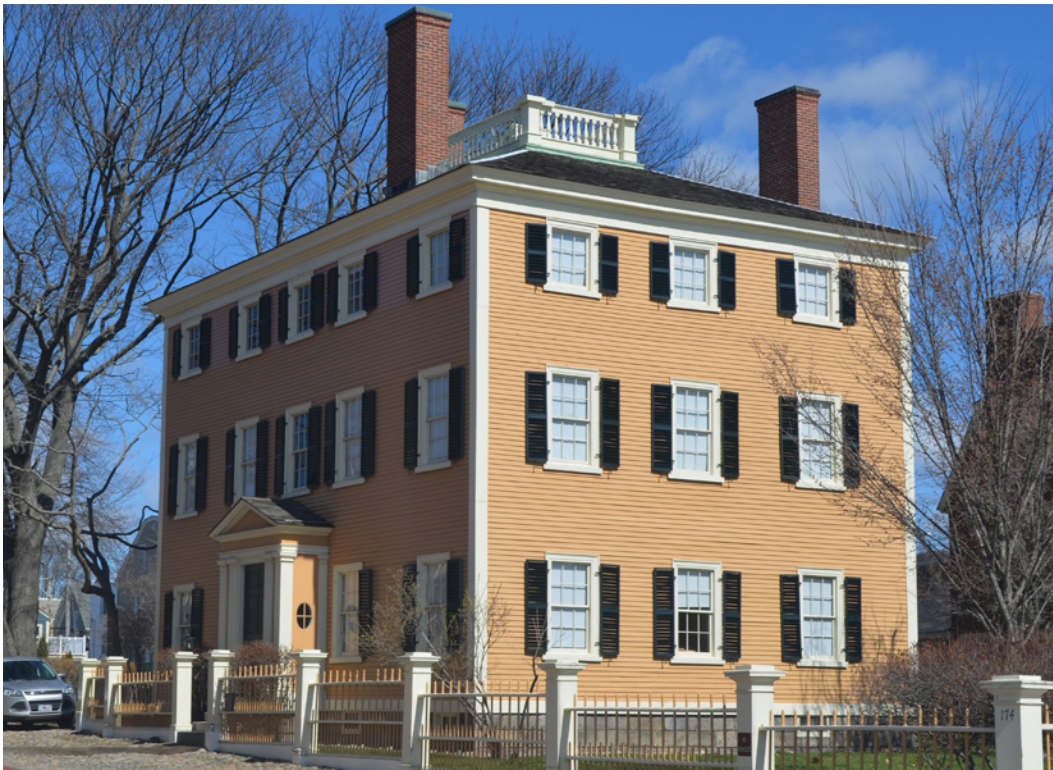
The Elias Haskell Derby-Benjamin Hawkes House (1780) is a well-preserved example of Federal style architecture in the Derby Street Historic District.
