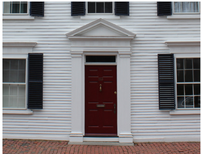
Georgian-Federal pedimented doorway, 6-panel wood door, simple single-lite transom, fluted pilasters and triglyphs.
