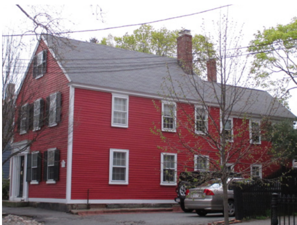
Example of a rear addition with setback facade and lower roof height, as well as continuity of materials and fenestration pattern matching the main building volume.
