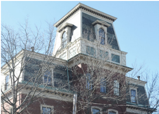
Slate shingles are common and prominent features of mansard roofs. Different slate colors and shaped shingles were often used to create decorative patterns.
