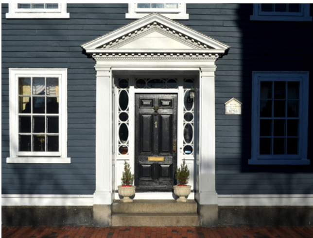
Pedimented door surround with fluted pilasters, 6-panel wood door, and hybrid tracery sidelights and transom.
