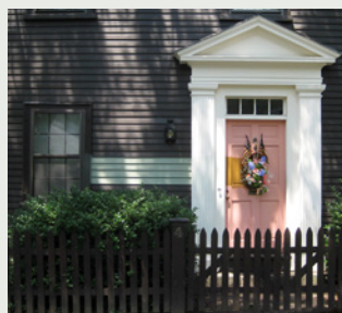
Example of physical color samples on the building.
