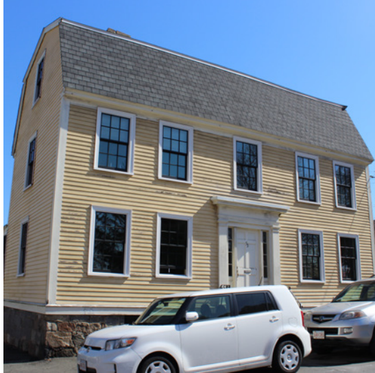
An example of approved replacement windows that fit the existing opening, maintain the original proportions, and have a historically appropriate multi-lite configuration.
