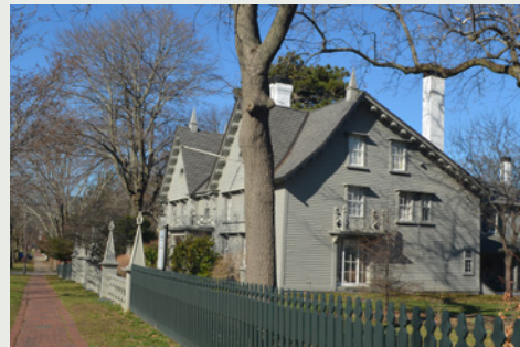
John Pickering House, 18 Broad Street. Full shot showing the existing conditions of the building's main and side facades.
