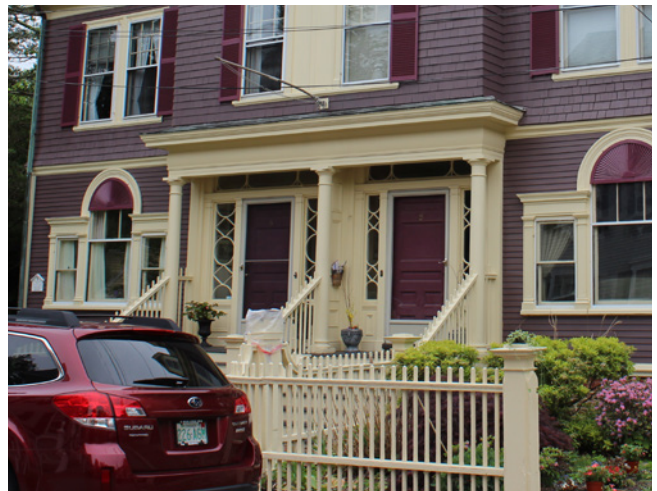
Colonial Revival double entry, multi-panel wood doors, large sidelights and transoms, and classical-style portico with narrow columns
