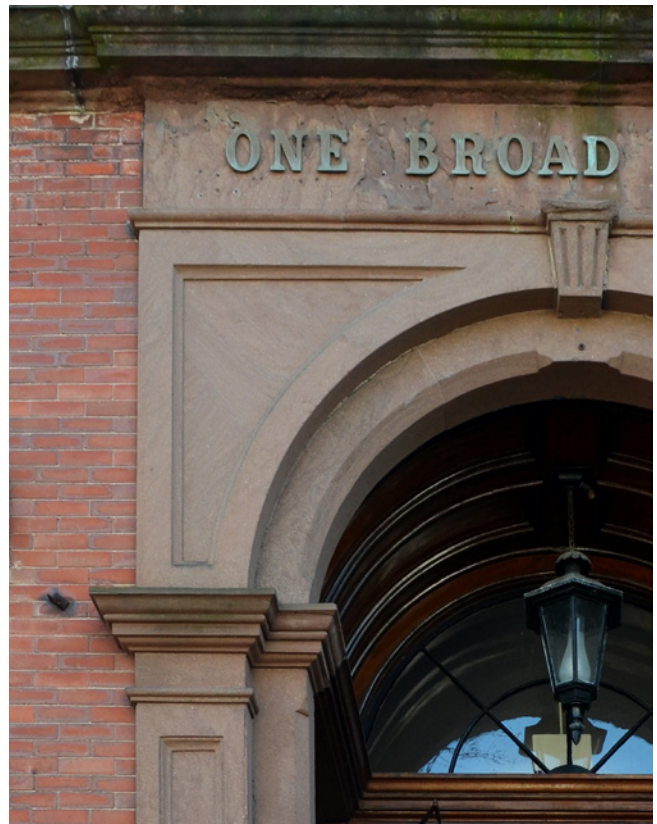
Details like sandstone entries, window surrounds, and quoins should be preserved.
