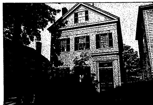
49 Summer Street is a fine Greek Revival building with flat board siding.
